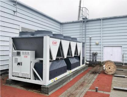
The AQUACIATPOWER chiller was lifted into position on the building within an enclosed courtyard.
