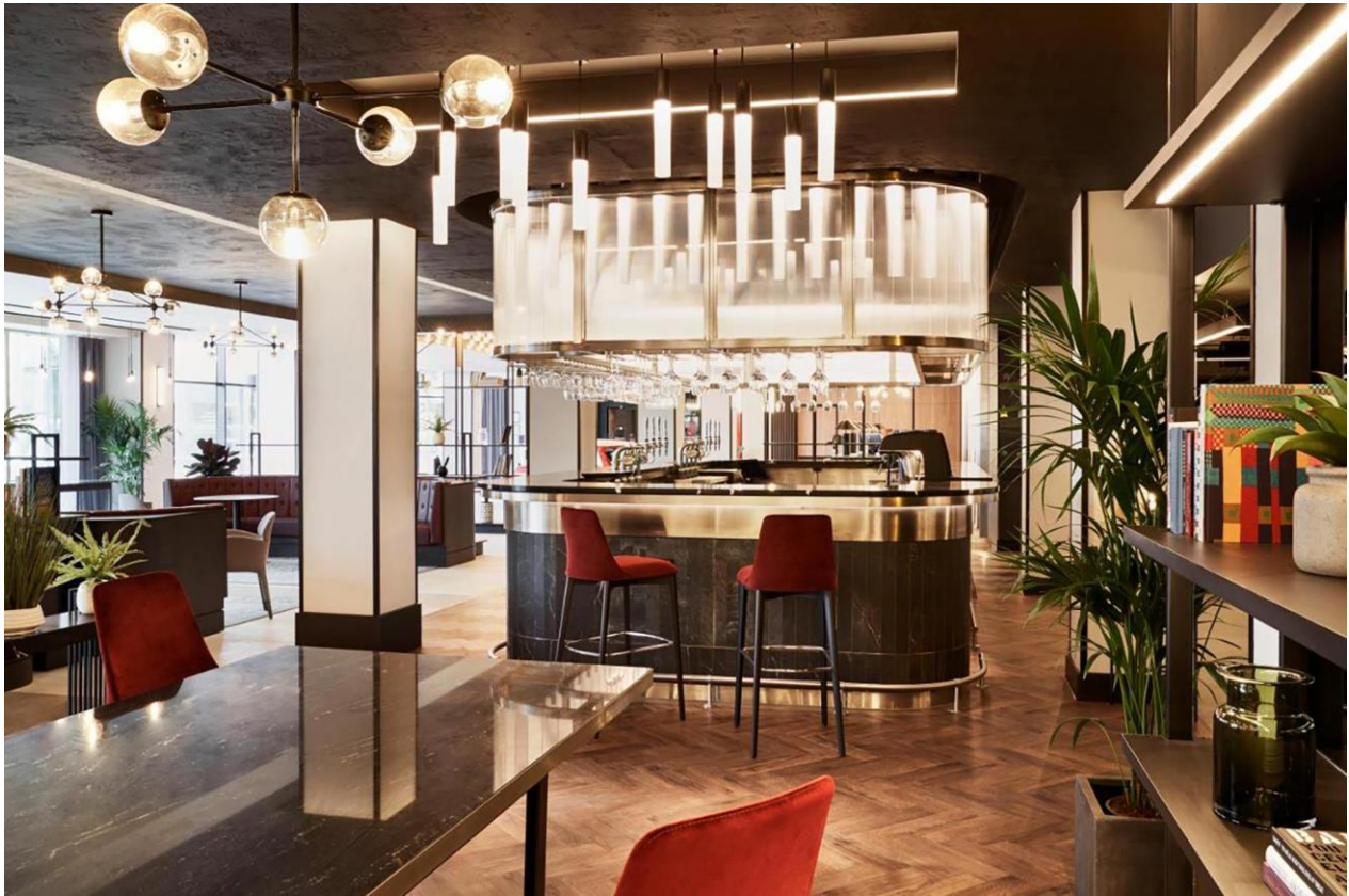
The new air conditioning system serves the hotel's bar and restaurant.
