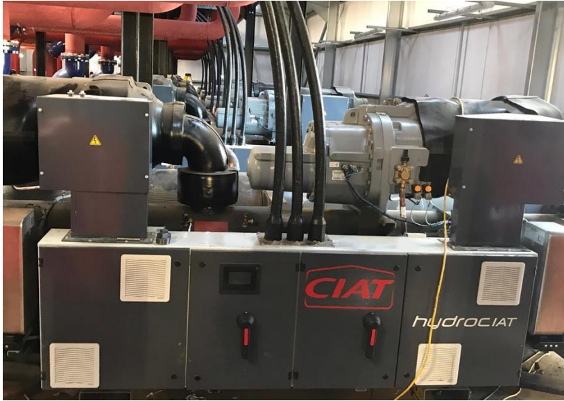
Left above: One of the five high-efficiency HydroCIAT heat pumps installed at the facility Right above: Pipework connecting the heat pumps to the rest of the system
