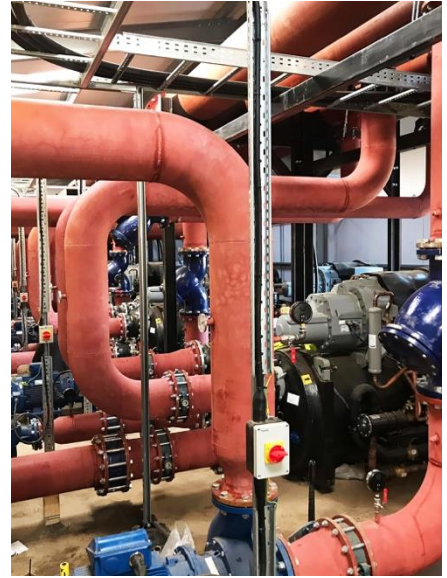
Left above: One of the five high-efficiency HydroCIAT heat pumps installed at the facility Right above: Pipework connecting the heat pumps to the rest of the system
