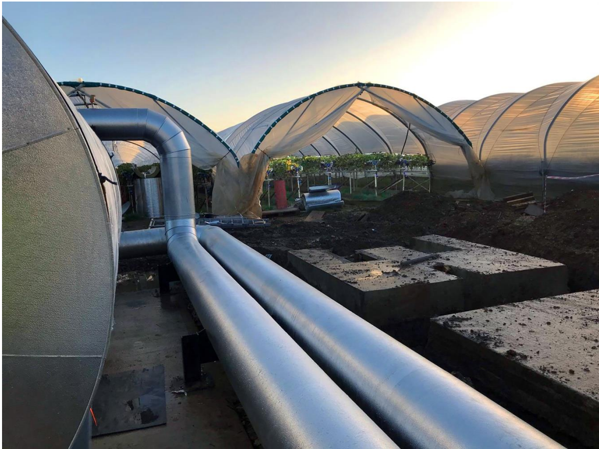
Growing tunnels full of produce are heated by the 8.8MW heat pump system
