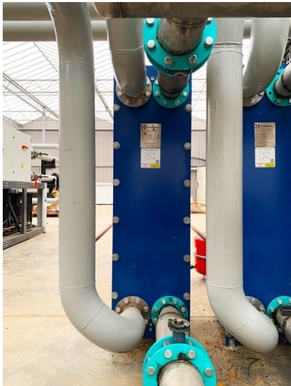
The system pumps ground-water from four abstraction boreholes up to 30m deep, passes it through the heat pumps to capture and upgrade its thermal energy.
