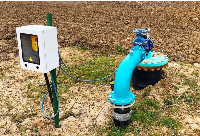
The system pumps ground-water from four abstraction boreholes up to 30m deep, passes it through the heat pumps to capture and upgrade its thermal energy.
